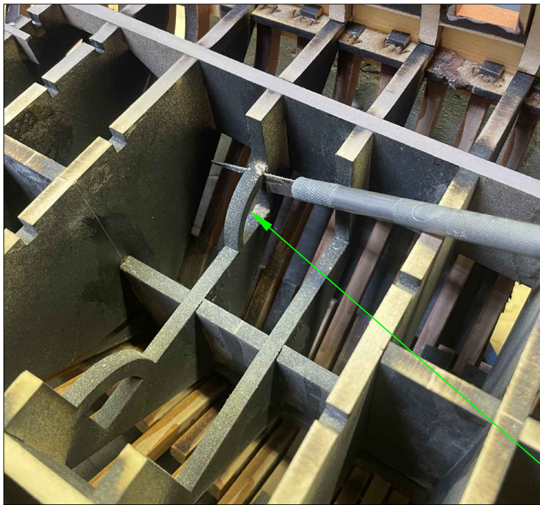
Aft orlop hoop supports being removed prior to orlop installation.
